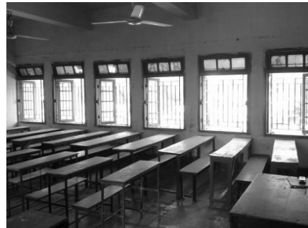
Figure 02: openings at north in classrooms
