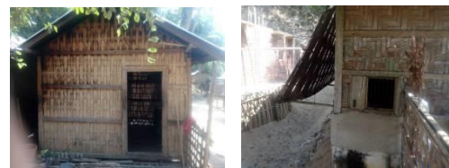
Figure 10: The wooden panelled door, the wall and the small windows
