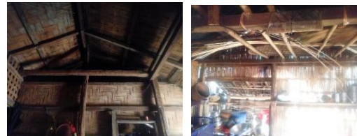
Figure 7: Use of beams in the roofing system (left) Space using in the beam (right)
