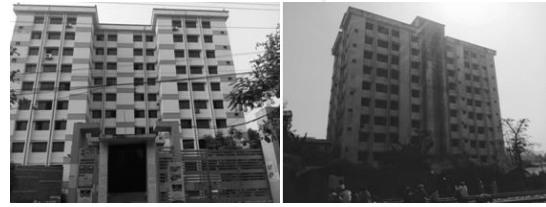
Figure 9: South and North side of the building
