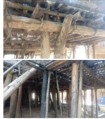
Figure 5: The bamboo joints with wooden post and bamboo post
