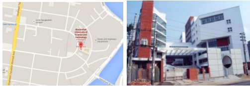
Figure 2: AUST with surrounding context.
