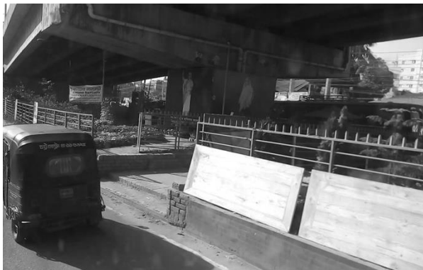
Fig. 04: Blow up of Bahaddarhat flyover present condition (location 1)
