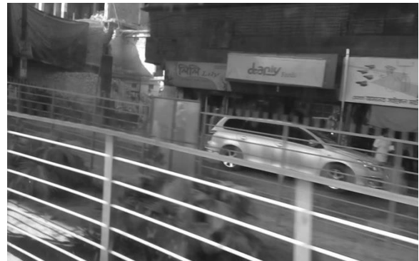
Fig. 07: Blow up of Bahaddarhat flyover present condition (location 4)
