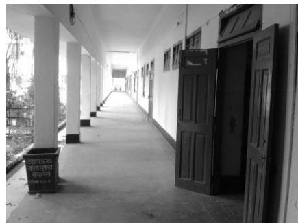
Figure 03: open corridor at south.
