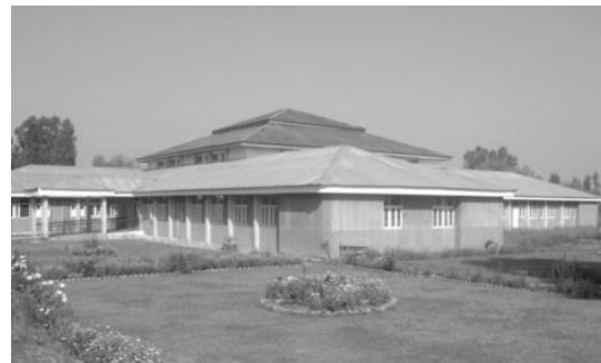
Figure 5 Exterior View of CRC, Srinagar
