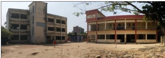
Figure 4: View from the open ground to the new building and the old building
