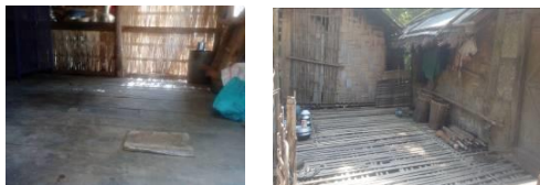
Figure 9: The wooden floor (left) and the bamboo fence floor (right)
