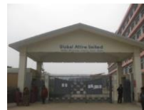
Figure 2: Front side of the case RMG building
