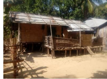
Figure 4: The bamboo fence around the open balcony.
