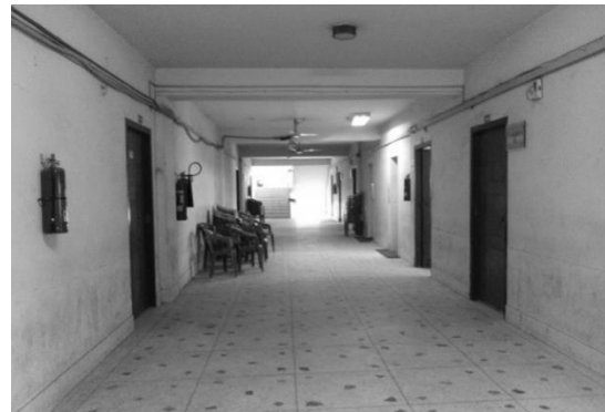
Figure 10: Central corridor of the building
