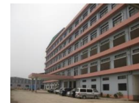
Figure 3: South elevation of the case RMG building
